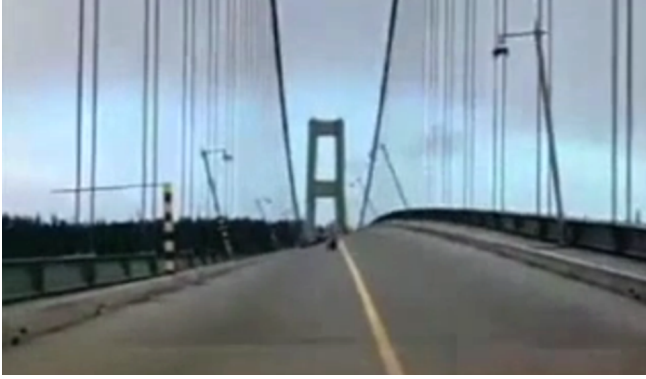
Figure 1. Empirical engineering in action: the first Tacoma Narrows bridge, oscillating torsionally just prior to its collapse. A simple optical instrument to measure the vertical displacement of the bridge deck can be seen on the left of the picture. The blurred figure near the centre line of the roadway is almost certainly that of Professor Burt Farquharson.
